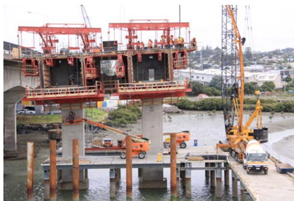
Manukau Harbour Crossing project (MHX) which will be completed August 2010.
