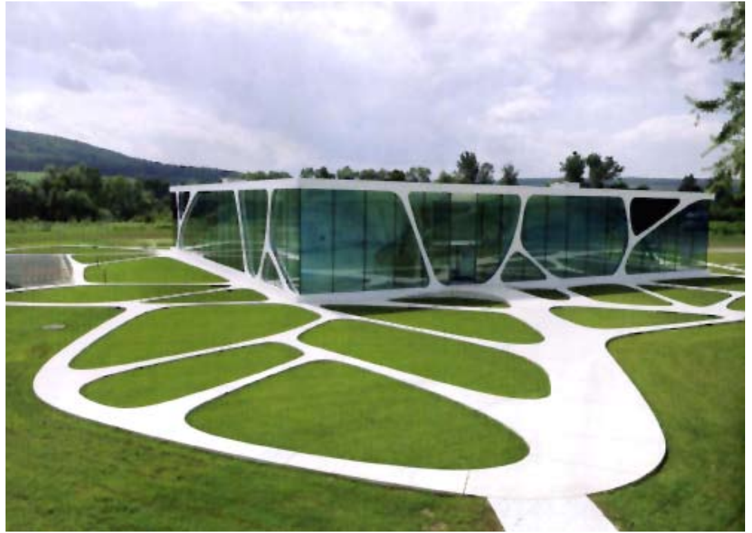
Glass Cube, European precast - striking image courtesy opus C - Concrete Architecture & Design
