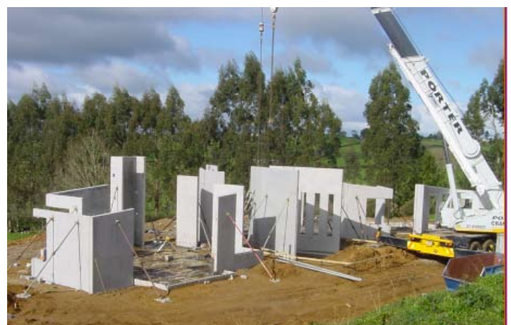
Litecrete residential panels being installed at Te Kowhai, Hamilton
